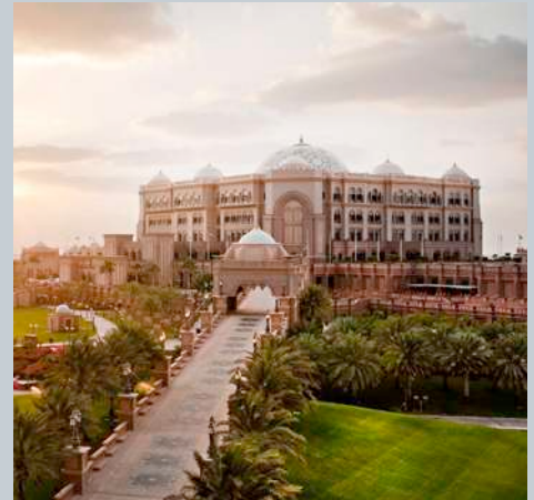
Emirates Palace Abu Dhabi
